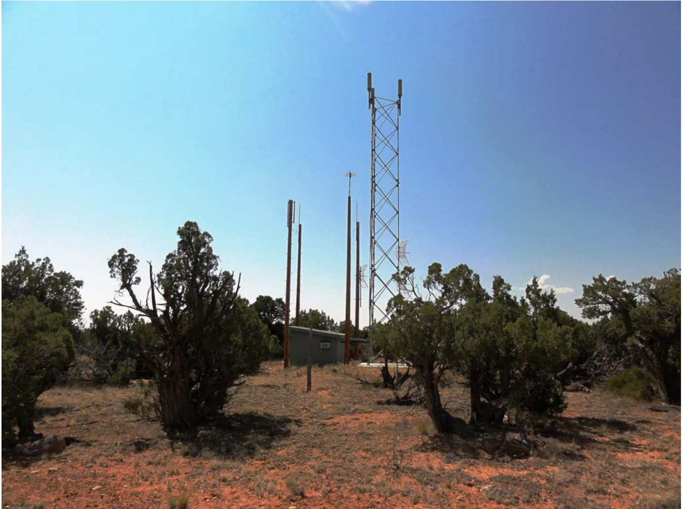
Photo 1- Existing Tower facility site looking southeast.
