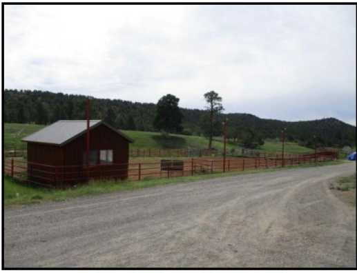
CORRAL WORKS AND LOAFING SHED
