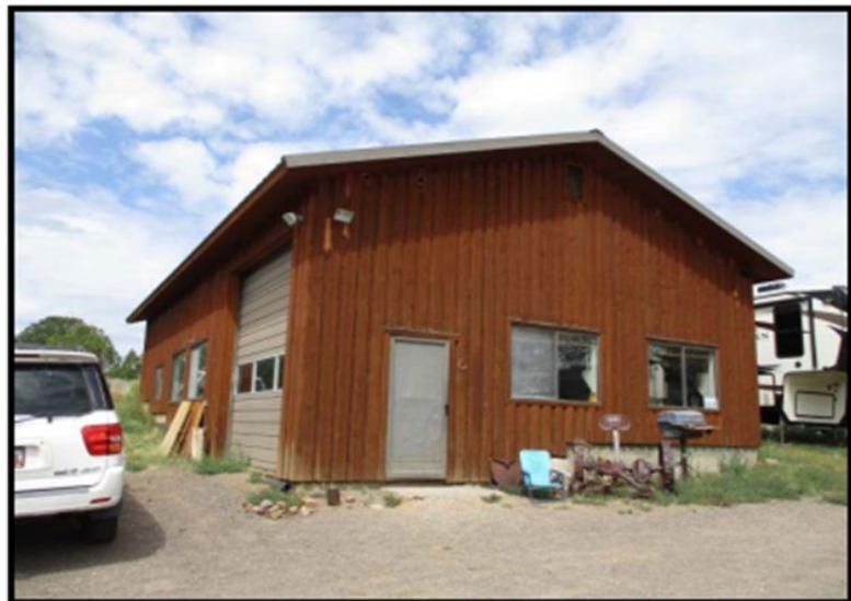
NORTHWESTERLY VIEW OF SHOP BUILDING
